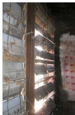
The photos depict the existing ("before") conditions typical at all six combustion air intake locations. The exterior (left) photo shows that the original fixed louvers and debris screen are no longer in place. They were removed at some time in the past, probably because they were not sized properly and could be blocked by a build-up of ice and snow. The interior (right) photo shows that many of the control arms linking the moving damper sections are either bent, broken, or missing.
