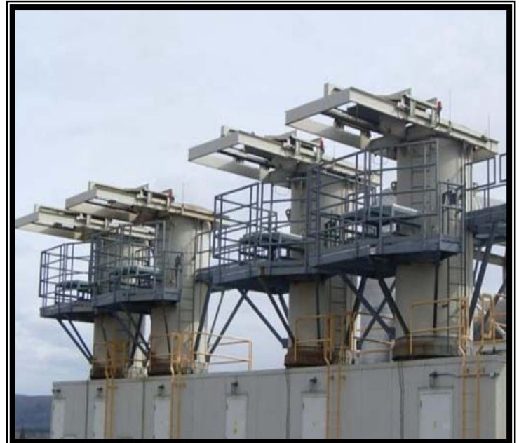
AFTER: New Boiler Stack Photo
