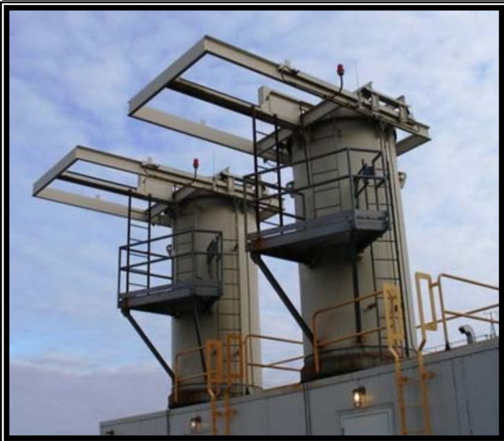
BEFORE: Old Boiler Stack Photo
