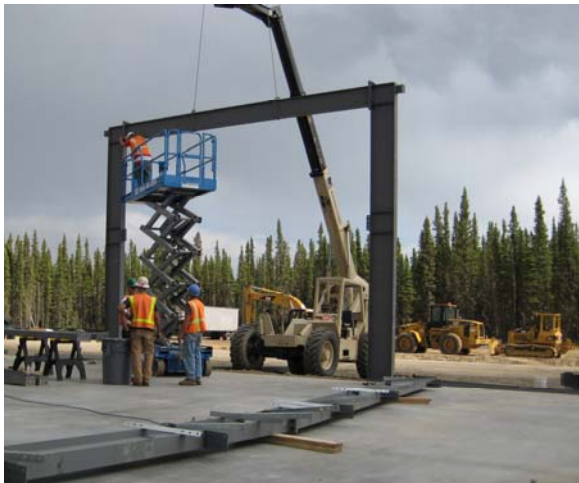
FGA Operations Depot being constructed
