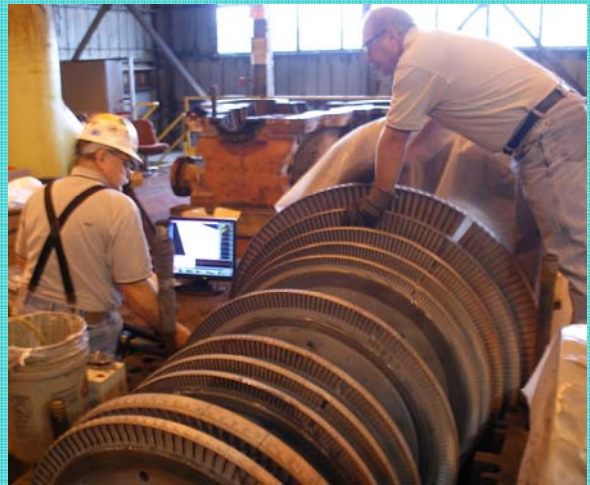
Photo above: A team of technicians conducts the phased array ultrasonic testing on the FWA CHPP Turbine #5 rotor.
