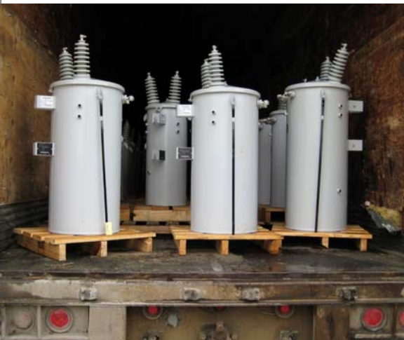
Transformers for feeders 5 & 9 being delivered
