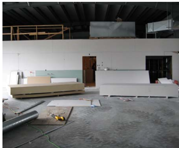
FRA Operations Depot— work on office space
