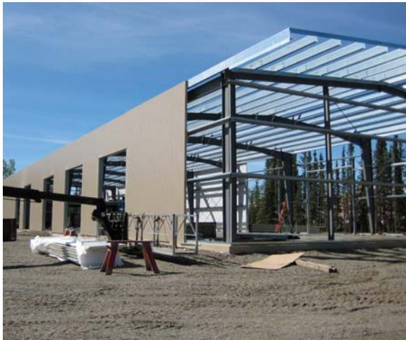
FGA Operations & Depot— outer walls going up
