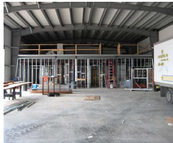
FRA Operations & Depot - offices being framed
