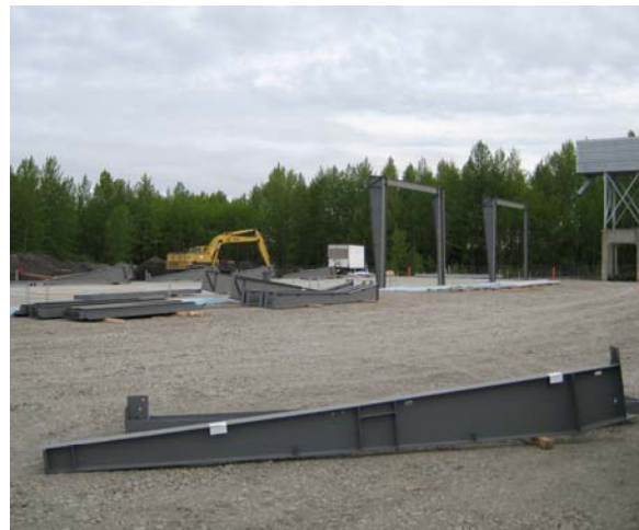
FRA Operations Depot with newly delivered steel
