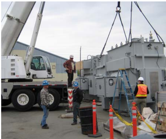
Placement of Transformer
