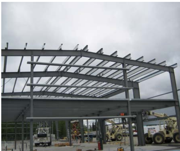
Steel continues to be erected for Ops Depot
