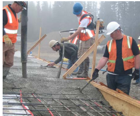
Concrete being poured at FGA Operations Depot Site
