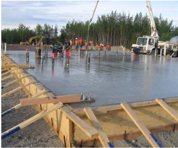
Concrete being poured at FWA Operations & Depot Site
