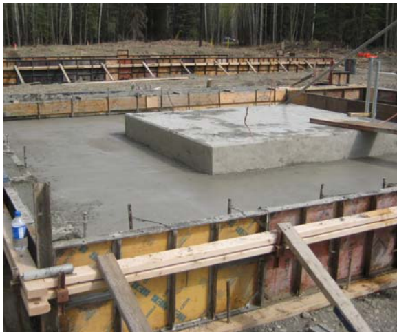
Substation Footings
