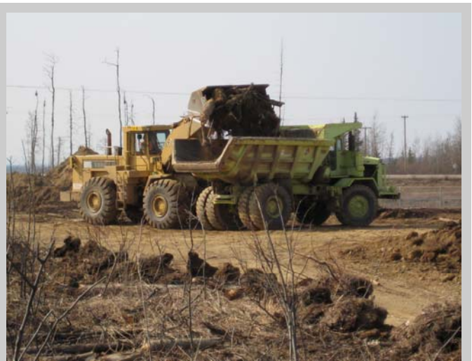
Picture (above): Clearing and grubbing at the Fort Greely substation site.
